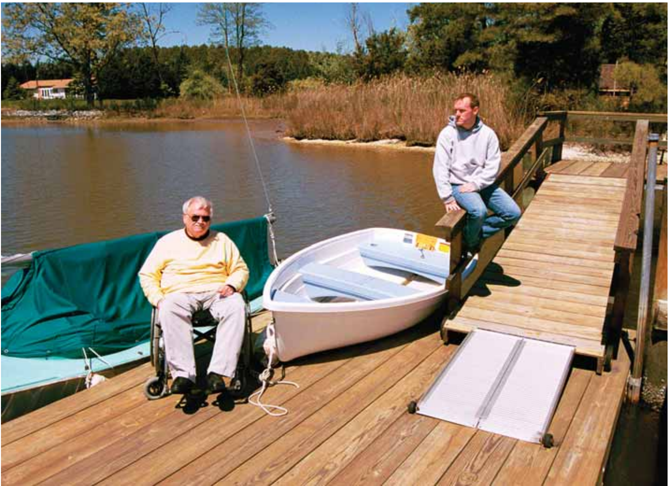
This floating dock rises and falls with the water level. The wood ramp and the metal transition edge are mounted on wheels to accommodate these fluctuations and the associated change in angle of incline.
